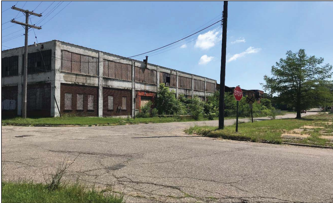
PHOTO NO. 1: View of building on the Property, looking northeast.
