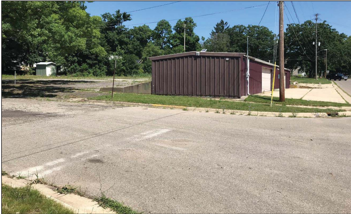
PHOTO NO. 17: View of the north-adjointing garage building.
