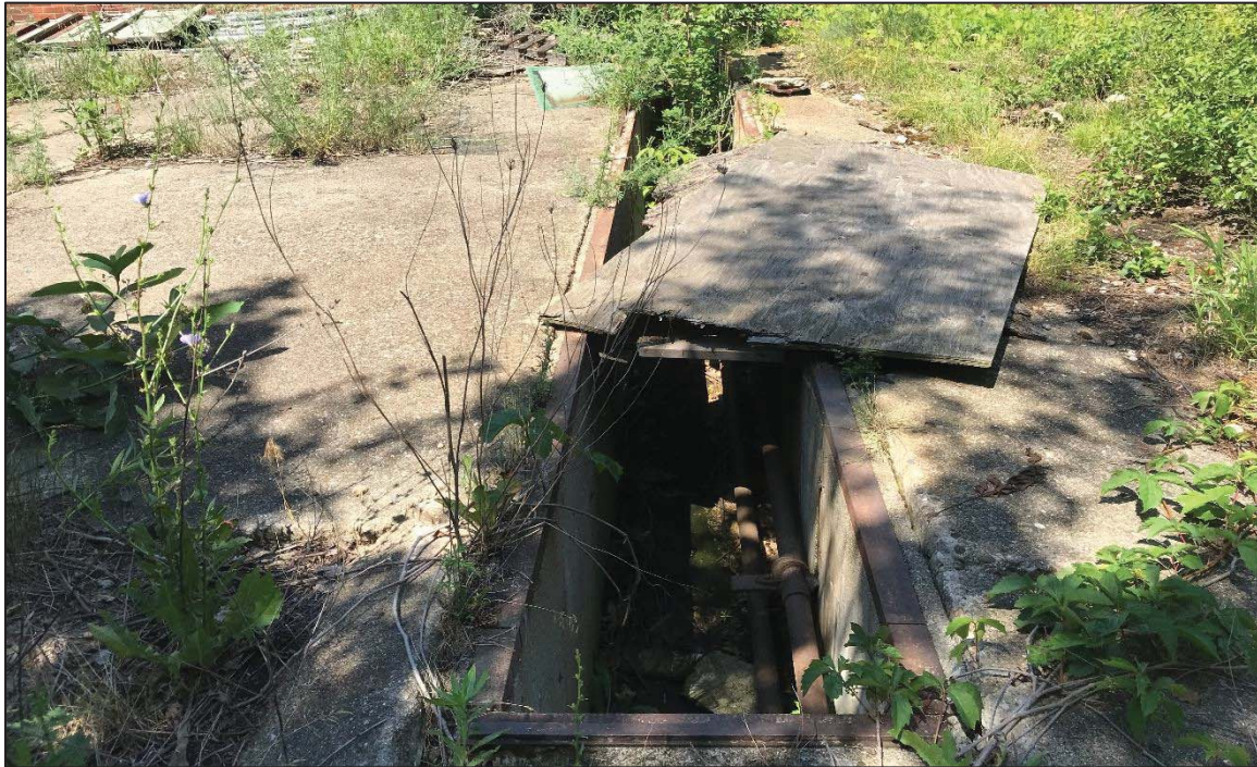
PHOTO NO. 11: View of a trench with piping and standing water observed in the eastern portion of the Property.
